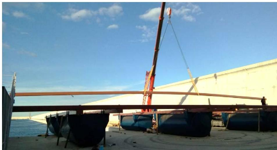
*Figure 50. Allocation of a secondary beam on the primary beams*
