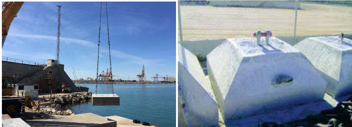
*Figure 59. Images of concrete anchors*
