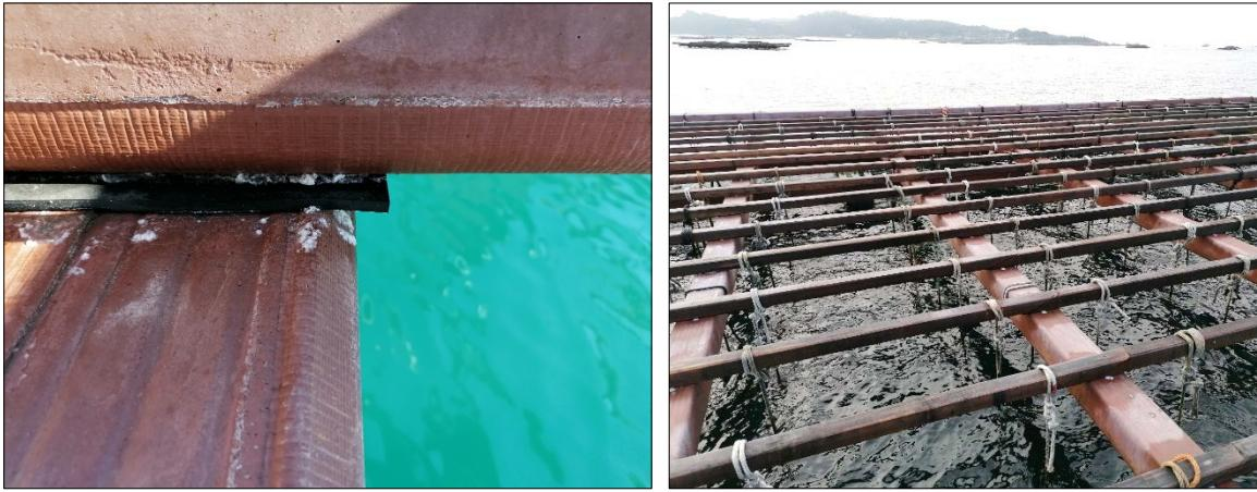
*Figure 41. Salt precipitation between two Formex® beams (left) and humid wooden joists due to the impact of the waves (right)*
