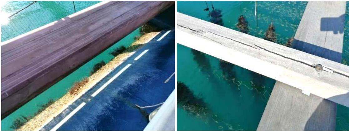
Figure 15. Floater with fouling (left). Right: Joist with a significant crack along its axis, generated by a screw
