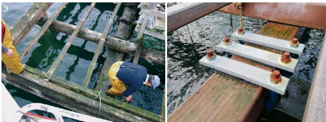
*Figure 17. “Verdín” in wooden beams (left) and in Formex® beams (right)*
