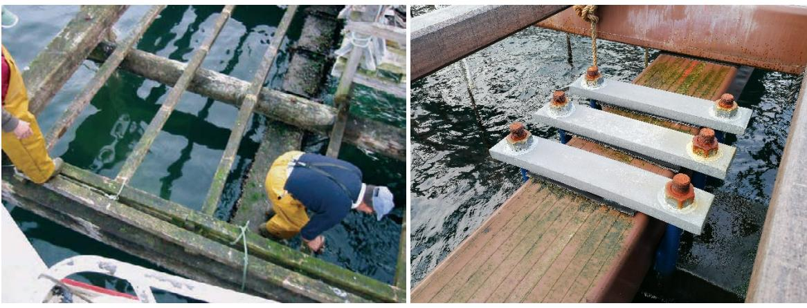
*Figure 40. “Verdín” in wooden beams (left) and in Formex® beams (right)*
