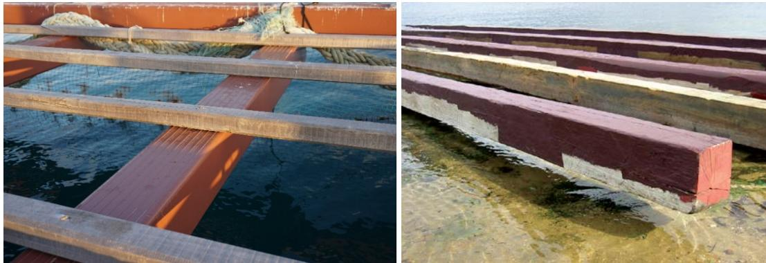
*Figure 32. Left: Primary beam in a Formex® raft. Right: Wooden beams protected with paint*
