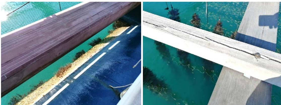
*Figure 33. Left: Floater with fouling in its surface. Right: Joist with a significant crack along its axis, generated by the screw*
