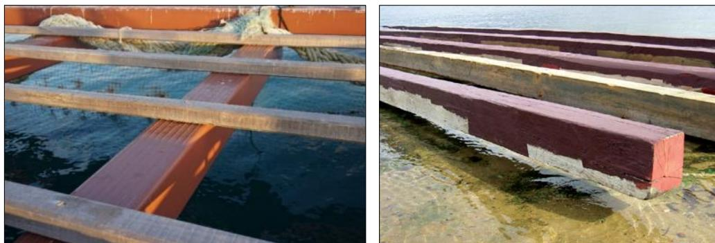
Figure 14. Left: Primary beam in a Formex® raft. Right: Wooden beams protected with paint
