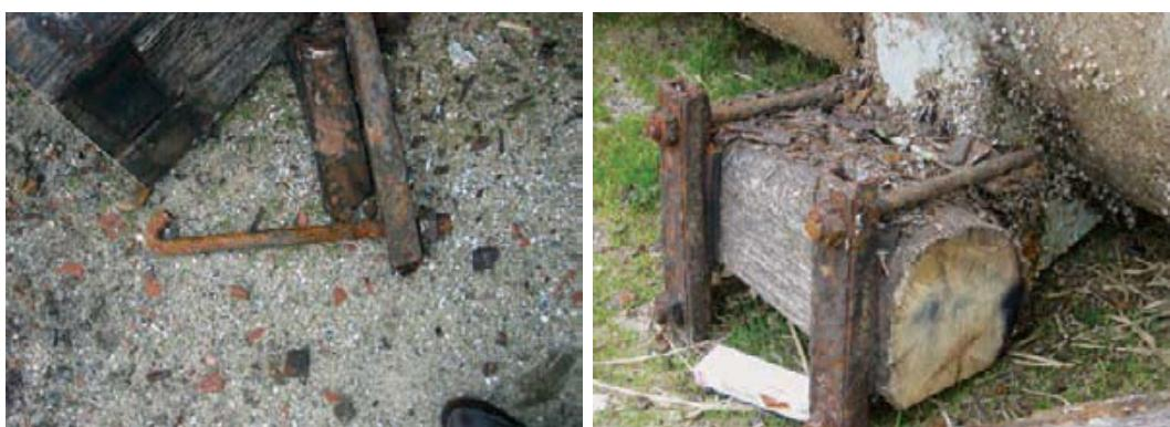
*Figure 35. Residues after an improper decommissioning of an old raft*
