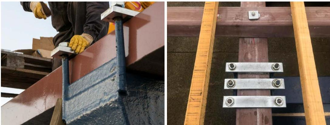
*Figure 44. Connection between the floater and a primary beam of a Formex® raft*
