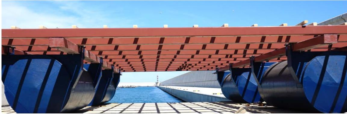
*Figure 55. Formex®Mixta raft after the installation of the joists*
