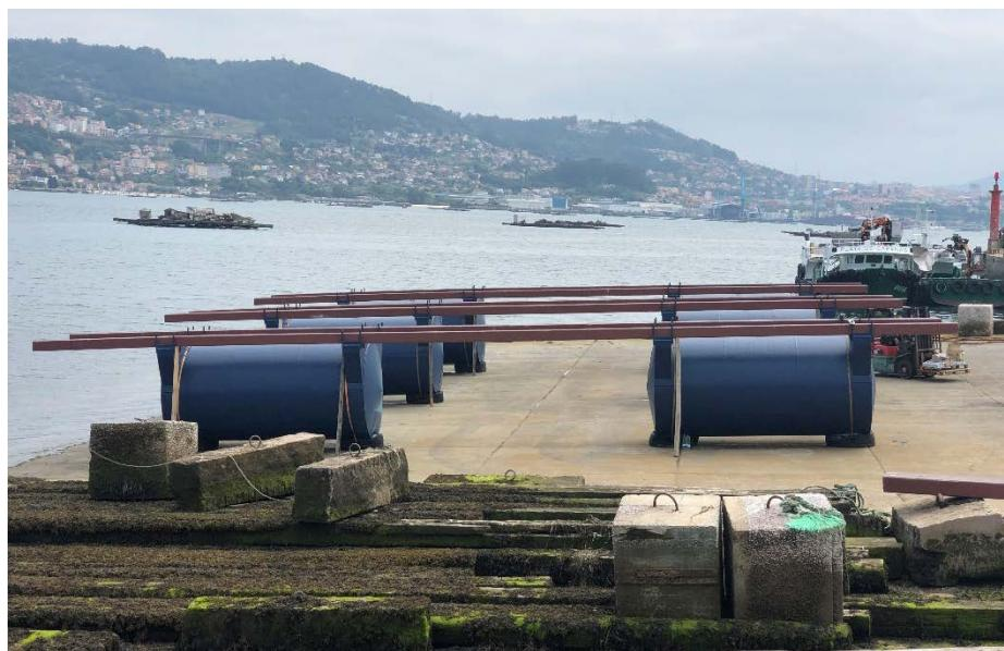
*Figure 48. Assembling of the primary beams in a Formex®Mixta raft*
