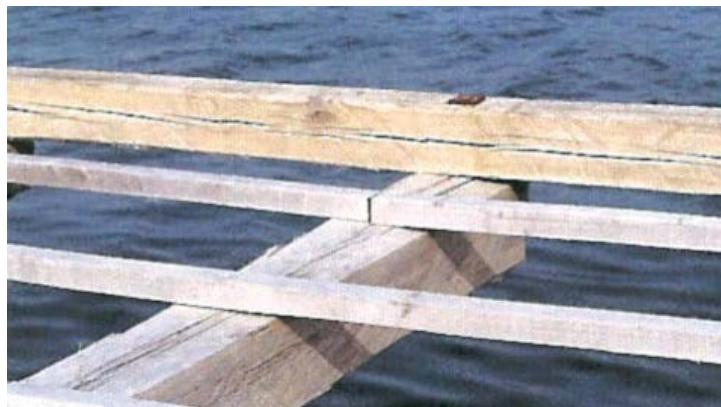
*Figure 52. Tie beam in a wooden raft. Figure 51 shows a tie beam in a Formex® raft*
