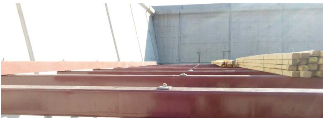
*Figure 51. Consecutive connections of the secondary Formex® beams along a primary Formex® beam*
