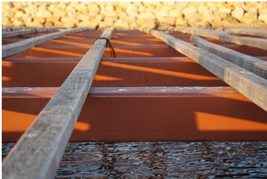
*Figure 26. Beams of a Formex® module. The corners are smooth and the surface is homogeneous*
