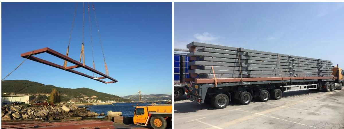
Figure 6. Left: Formex® frame adequately manipulated. The rigger uses a rope to guide the load and the weight is equilibrated using the required slings. Right: Truck with load appropriately trimmed
