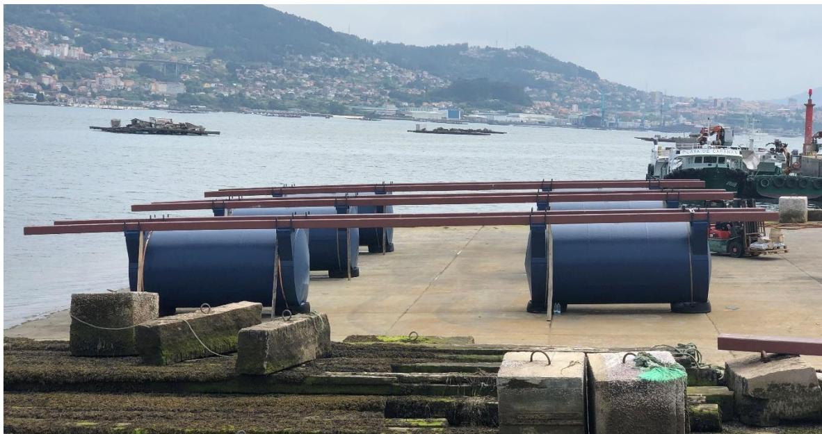
*Figure 12. Positioning of the floaters and primary beams of a Formex® Plus raft in a ramp. Low tide.*
