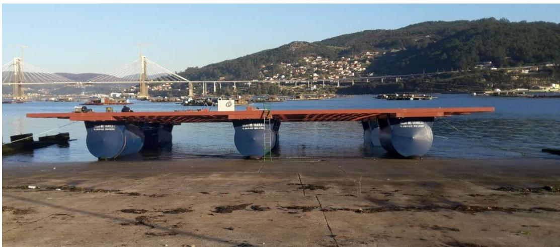
*Figure 13. Raft assembled one and a half day after starting the work. Tide is starting to rise*
