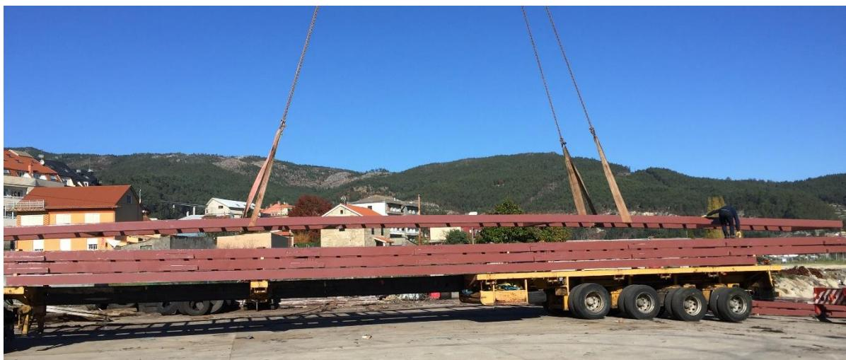
Figure 7. Formex® frame being lifted slowly to verify the equilibrium of the loads before staring the process
