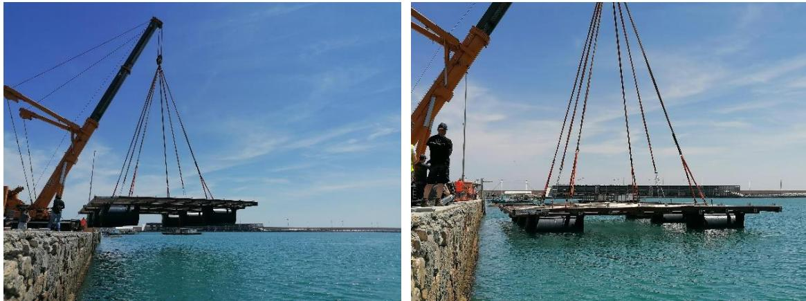
*Figure 11. Sequence that shows the floating of a Formex® raft in Valencia port for the H2020 project ReSHEALience-760824*
