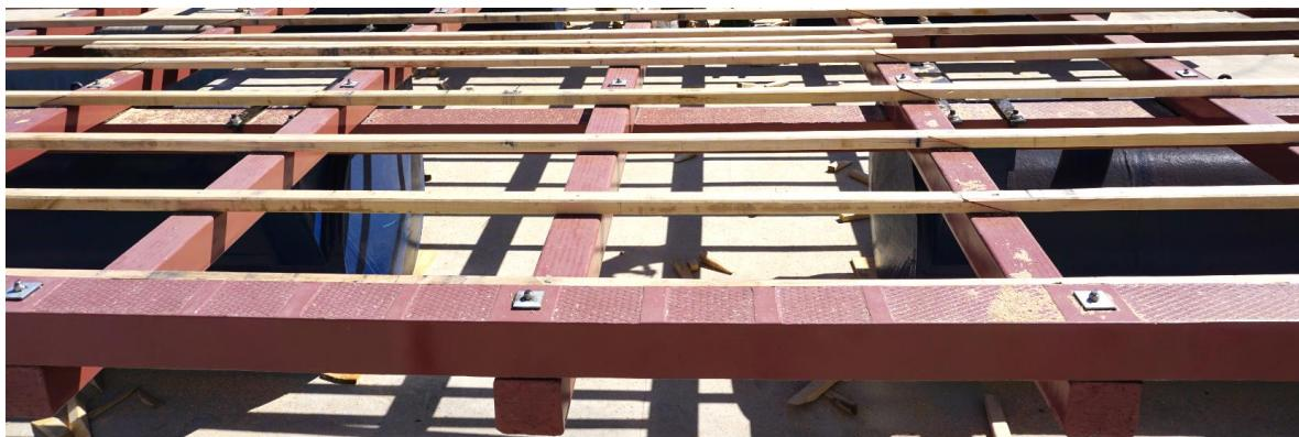
Figure 31. Adequate connection between the perimetral beam and the secondary beams. It can be seen that the thread is at the top side
